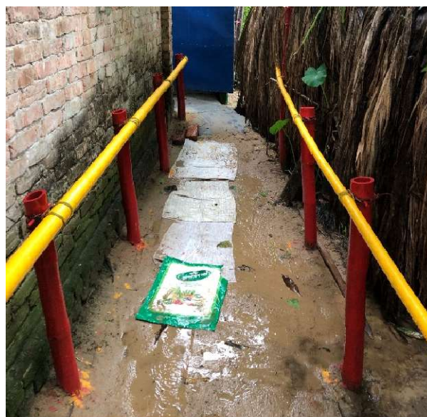
Handrails out of bamboo canes are colored in red and yellow for visibility. ©CBM UK
