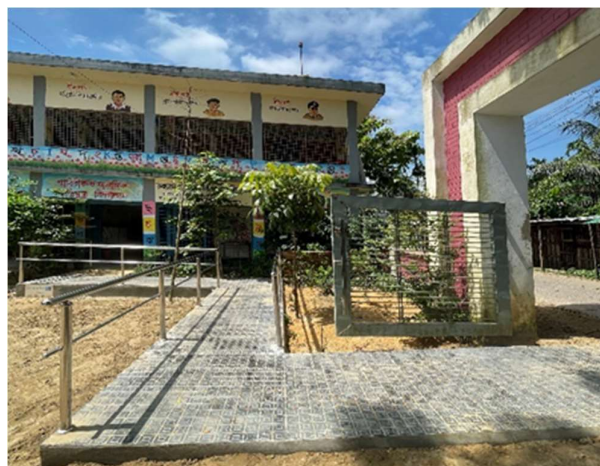
Handrails and a wheelchair ramp were installed at a primary school in Cox's Bazar. ©CDD Bangladesh
